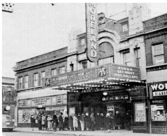
The old Moreland Theatre on Buckeye Road
